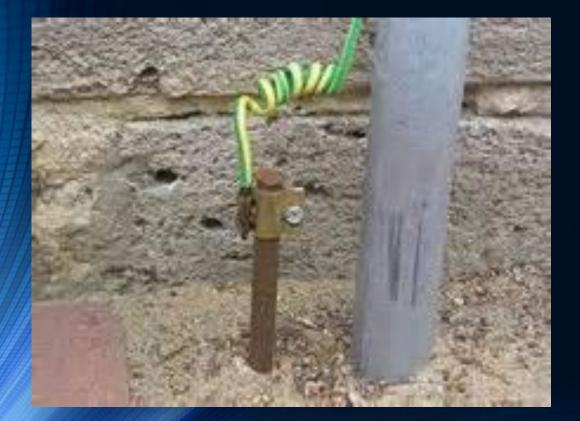
Allowing charges to flow directly from the circuit into Earth in the event of a short circuit.
